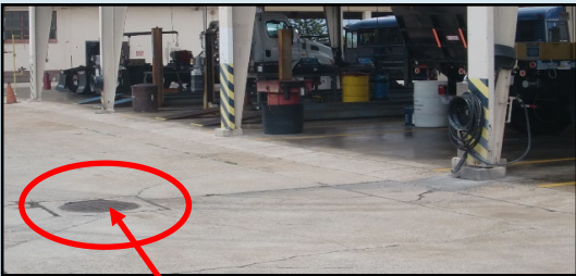
Photo: An unprotected storm drain inlet, located downstream of work areas, is a critical area to protect from potential pollutants.
