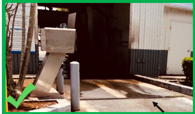
Photos: (Top) Overspray leaving wash bay. (Bottom) Sump drain system collects wash water overflowing from wash bay for treatment.
