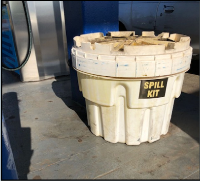
Photo: Clearly labelled spill kit stored beside fuel pump.
