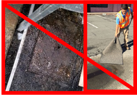
Photos: (Left) Inadequate maintenance of a grease trap can lead to overflows of wastewater, food waste, oil, and grease. (Right) Improper disposal of rinse water to a nearby storm drain inlet.
