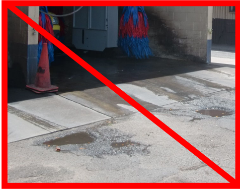
Photo: Wash water overflowing out of wash bay to parking lot.
